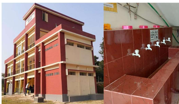
Fig. 9 (L): Constructed Wash Block (R): 5 outlet water collection basin
